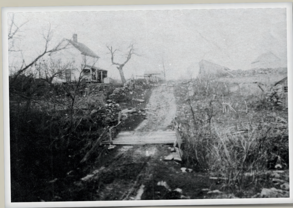
Whitman Farm, Road, and Bridge
