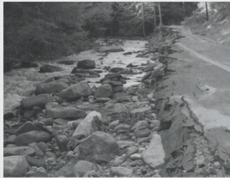
Pine Kill Road Washout of 2004
