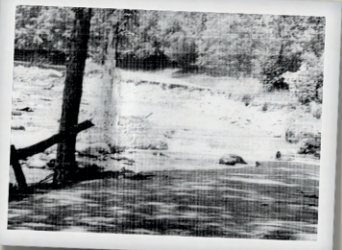
Washout of the Pine Kill Road
